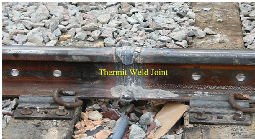
Fig. 2. Thermit joint Weld [17].
