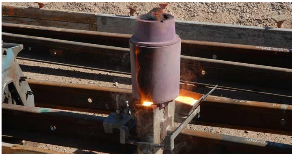
Fig. 1. Thermit railway welding [15].
